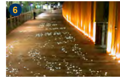
6 LED Fibre Optics inset into pavement
