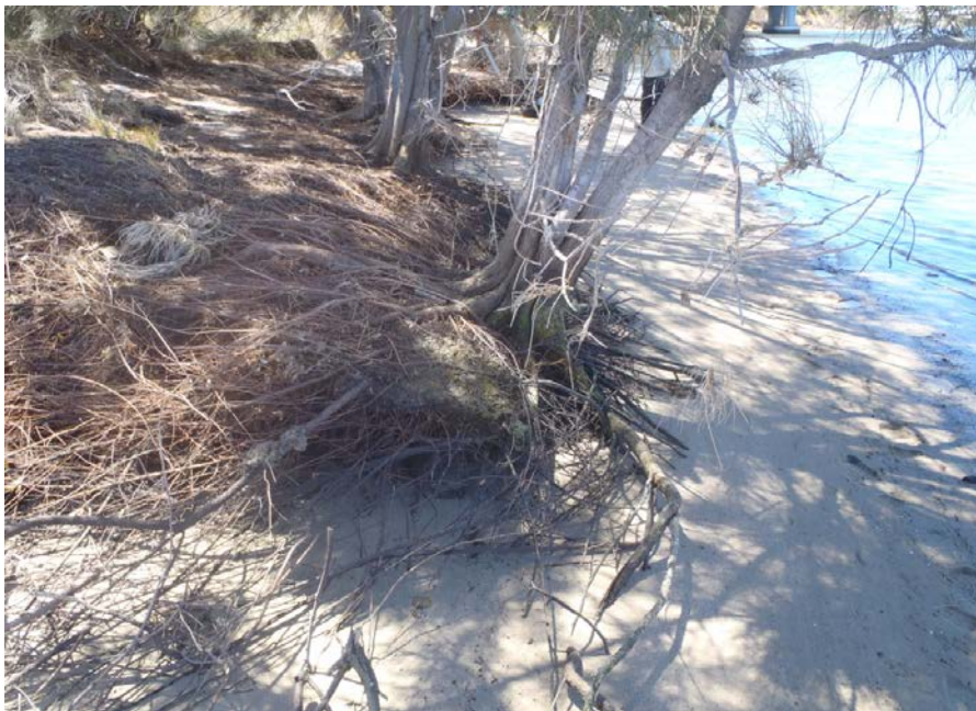
Figure 17 Foreshore treatment 2 restoration area – south western foreshore
