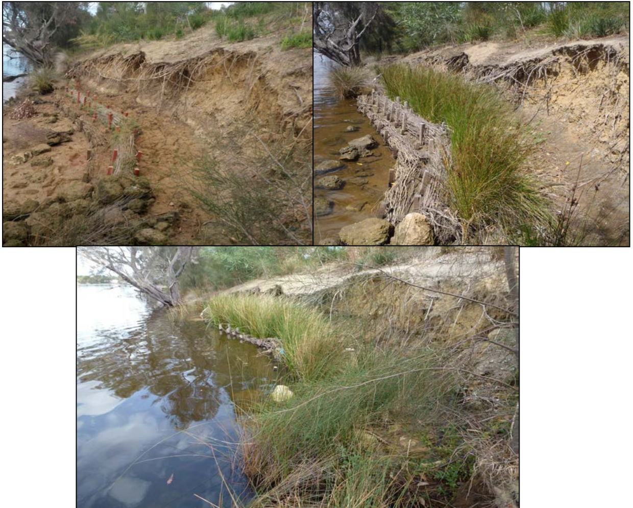
Figure 15 Brushwall examples prior to and after plant establishment and during high tide (Source: Syrinx, 2013)
